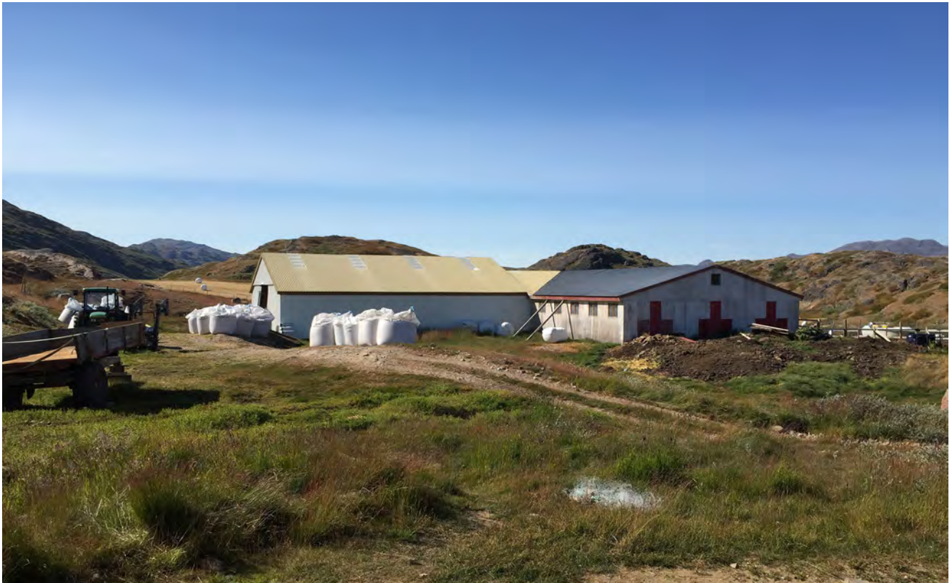
Fig. 2.126: Wooden shed from the late 1980s and a steel barn from the 1990s at the Tasilikuloq farm.
